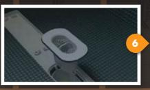
Spread the adhesive evenly over the area where the shower tray is to be installed, being careful to clean away any adhesive on the rim of the trap.
