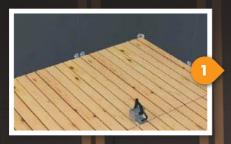
Put shower tray in the correct position and mark around the tray, to establish which section of the floor boards needs to be removed, the tray can be recessed.
