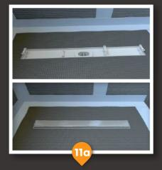
If you're not using a tile on grate, adjust the height of the stainless steel support utilising the height adjustment spacers, each space will increase the height by 1.5mm.
