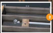
Once the floorboards are removed, measure and mark where your drain and waste pipe will be fitted. Please note: The drain body needs to be split into 2 parts, the upper part fits to the underside of the former and the main body goes into the floor.
