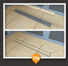
If you're using a tile on grate, the height of the stainless steel support can be adjusted utilising the height adjustment spacers, but the inner height of the tile on the grate is fixed (13mm). Please ensure that you use suitable tiles for the grate and the shower tray.
